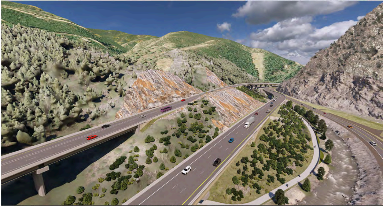
I-70 AND SADDLE CUT LOOKING WEST
